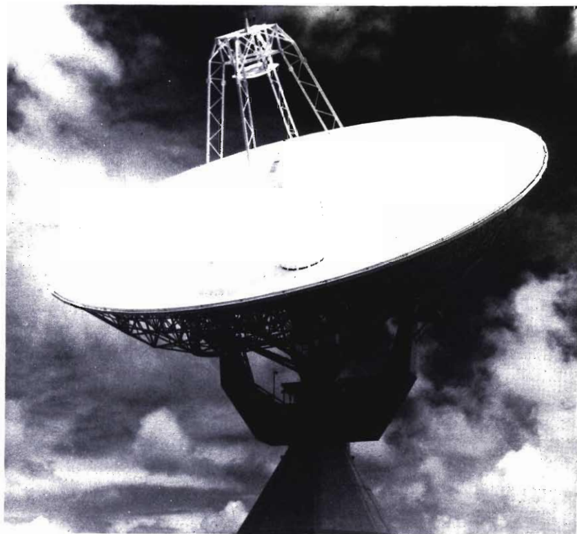
Fig. 6 THIS 85-FOOT ANTENNA is located at a COMSAT earth station and is used to relay high speed communication data between North America and the Far East via the Pacific satellites. This is one of six U.S. earth stations used to handle international communications. Imagine how a comparable dish antenna like this would work on the CB channels! Any takers?
